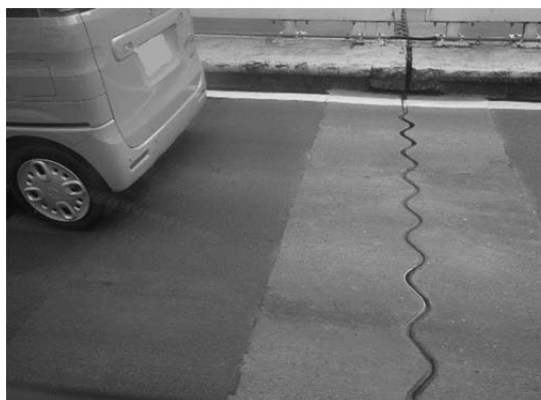
Fig. 1 Expansion joint on expressway
