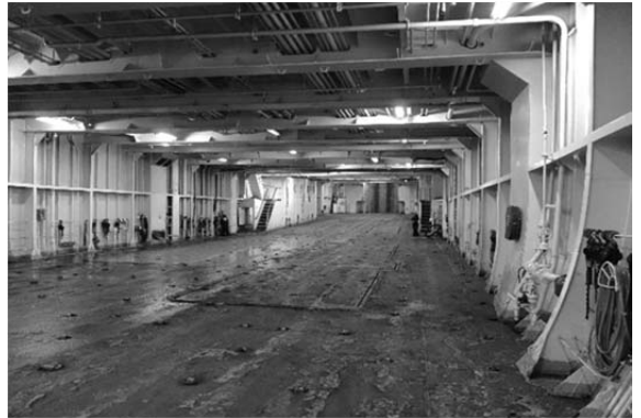
Fig.15 Floor surface with a lot of brackets.
