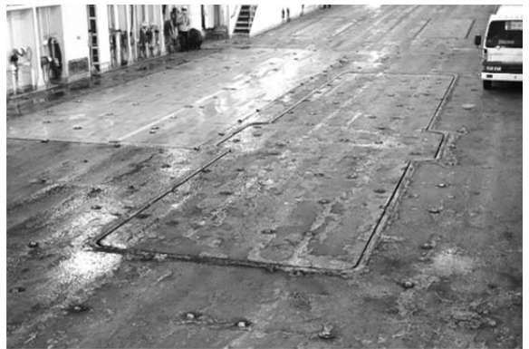
Fig.16 Floor surface with rough surface
